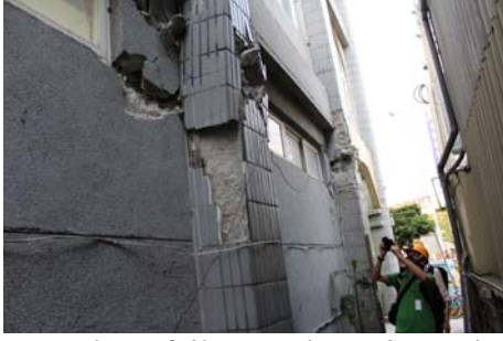
Figure 6. Shear failure and gravity resistance loss of an extremely short column.
