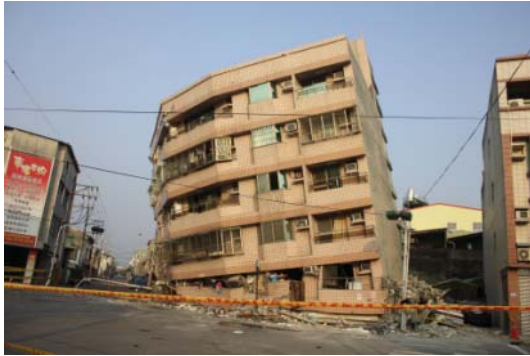
Figure 8. Buildings at the corner of an intersection collapsed in 0206 Meinong Earthquake, owing to eccentric rotation
