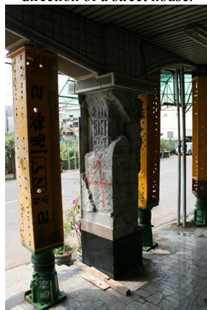
Figure 5. A corridor column with non-ductile detailing.
