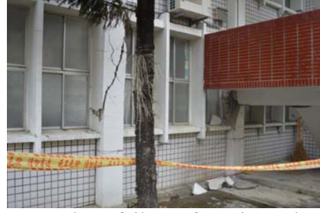
Figure 7. Shear failure of captive columns.
