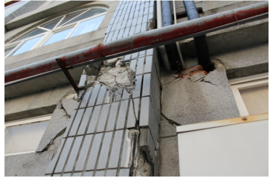
Figure 9. Shear failure of short columns in high windows
